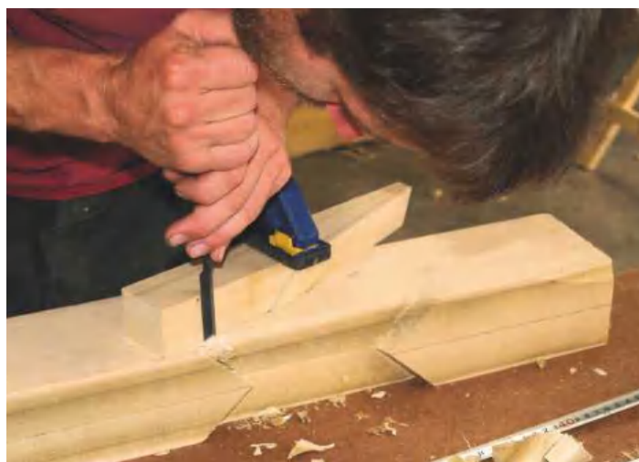
▲ Pic.16 Using a paring guide for the shoulders of the oblique lap cut on the underside of the hip
